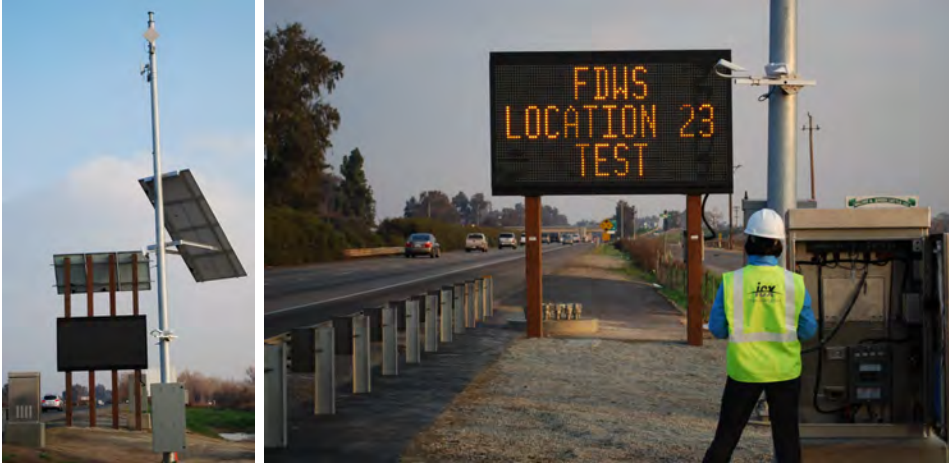
Figure 3.1: CalTrans Fog Detection and Warning System [19].
