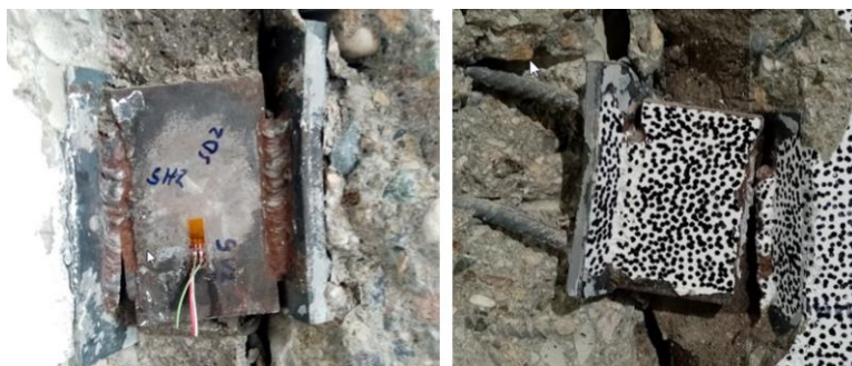
Figure 3-5 Welded plates after failure (1st test vs 3rd test)
