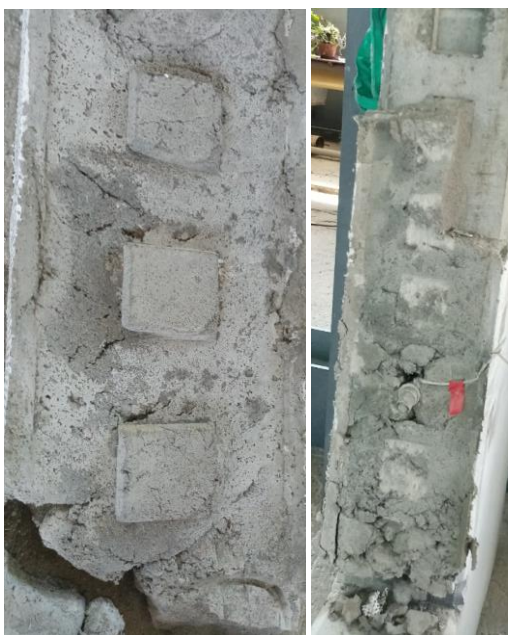
Figure 3-35 Observed grout quality after testing (SA3T3)
