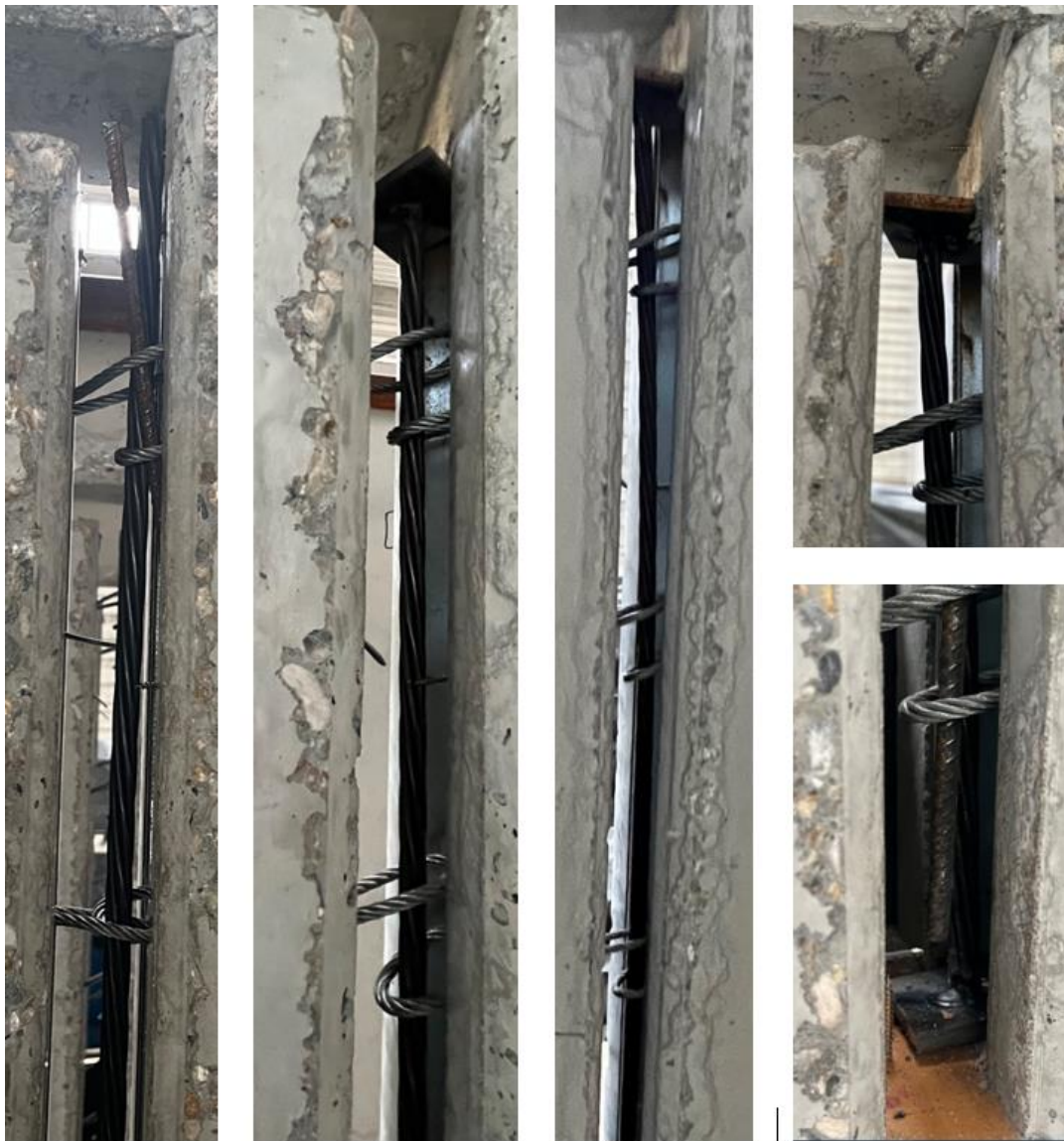
Figure 4-40 Test specimens before joint casting
