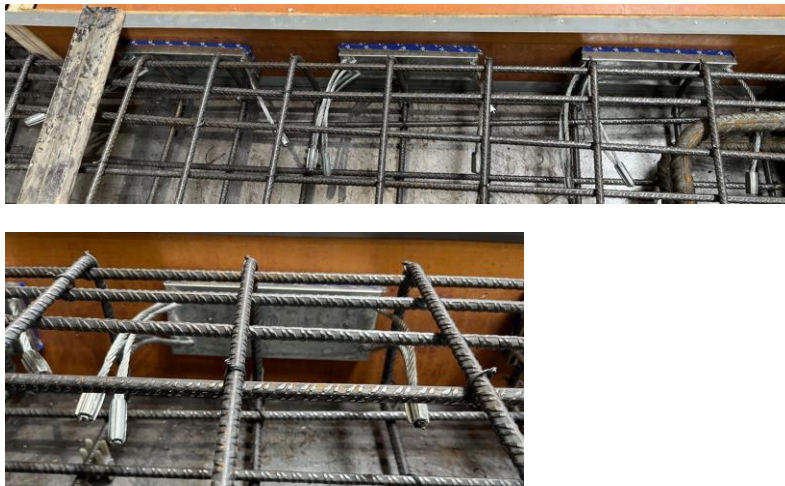
Figure 4-32 Wire boxes before panels casting
