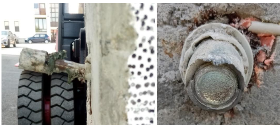
Figure 3-33 Part of the bolted steel assembly in the grouted area
