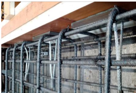
Figure 4-3 Wire boxes before panels casting
