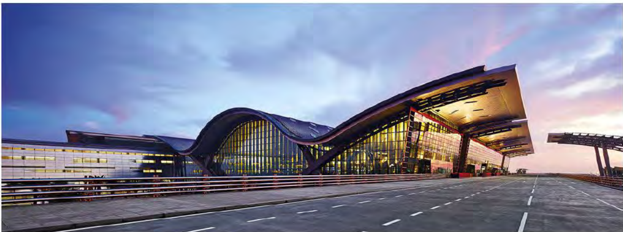
Hamad International Airport in Doha, Qatar has a duplex stainless steel roof. © Hamad International Airport
