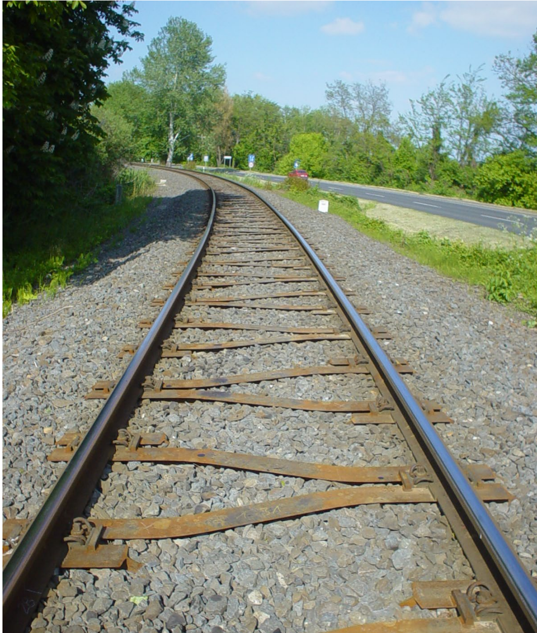
Figura 2.13 Tronson experimental cu traverse metalice tip Y, Ungaria
