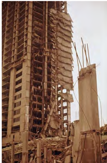
Figura 11. Eșecul The skyline plaza apartment BUILDING
