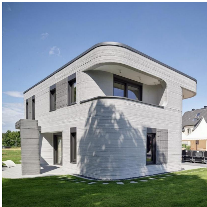
Figure 9. Full-size house realized via 3D printing [41].
