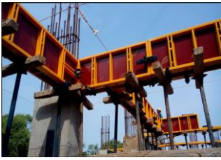
Formwork and support
